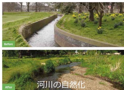
Figure 2.27. The Braid Burn, Edinburgh, before and one year after work to lower an artificial raised bank and replace the concrete channel with sinuous meanders: This work formed part of wider flood alleviation works carried out by the City of Edinburgh Council that sought to also improve biodiversity and public amenity on this watercourse (© River Restoration Centre).
