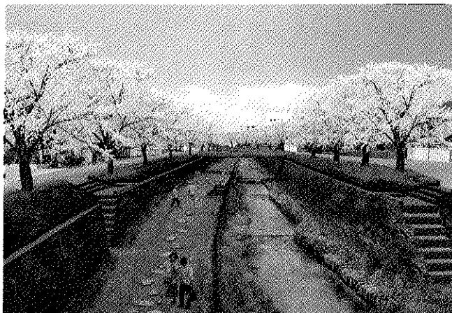
写真4 高水敷を片側に寄せ、沿川植樹の樹種はソメイヨシノとする Photo 4 High-water channel placed along one bank, with Somei Yoshino cherry selected as the tree species to be planted along the river
