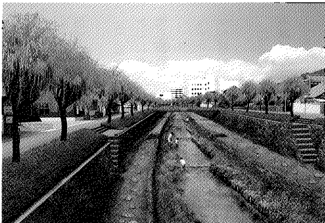
写真2 両岸に高水敷を設け、沿川樹木の樹種はシダレヤナギとする Photo 2 High-water channels placed on both banks, with weeping willow selected as the tree species to be planted along the river
