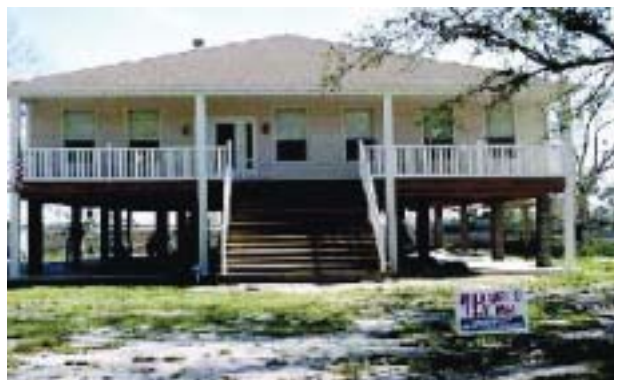
図-6 Elevation(open foundation)の例(FEMA資料)
