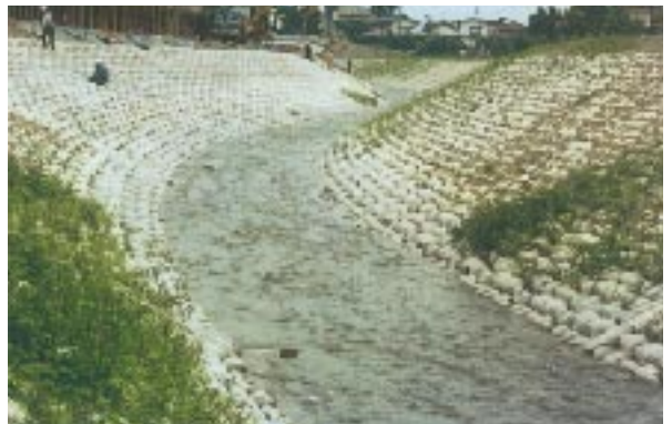
写真7 2割勾配の護岸を有し低水路幅が狭い河道の事例2
